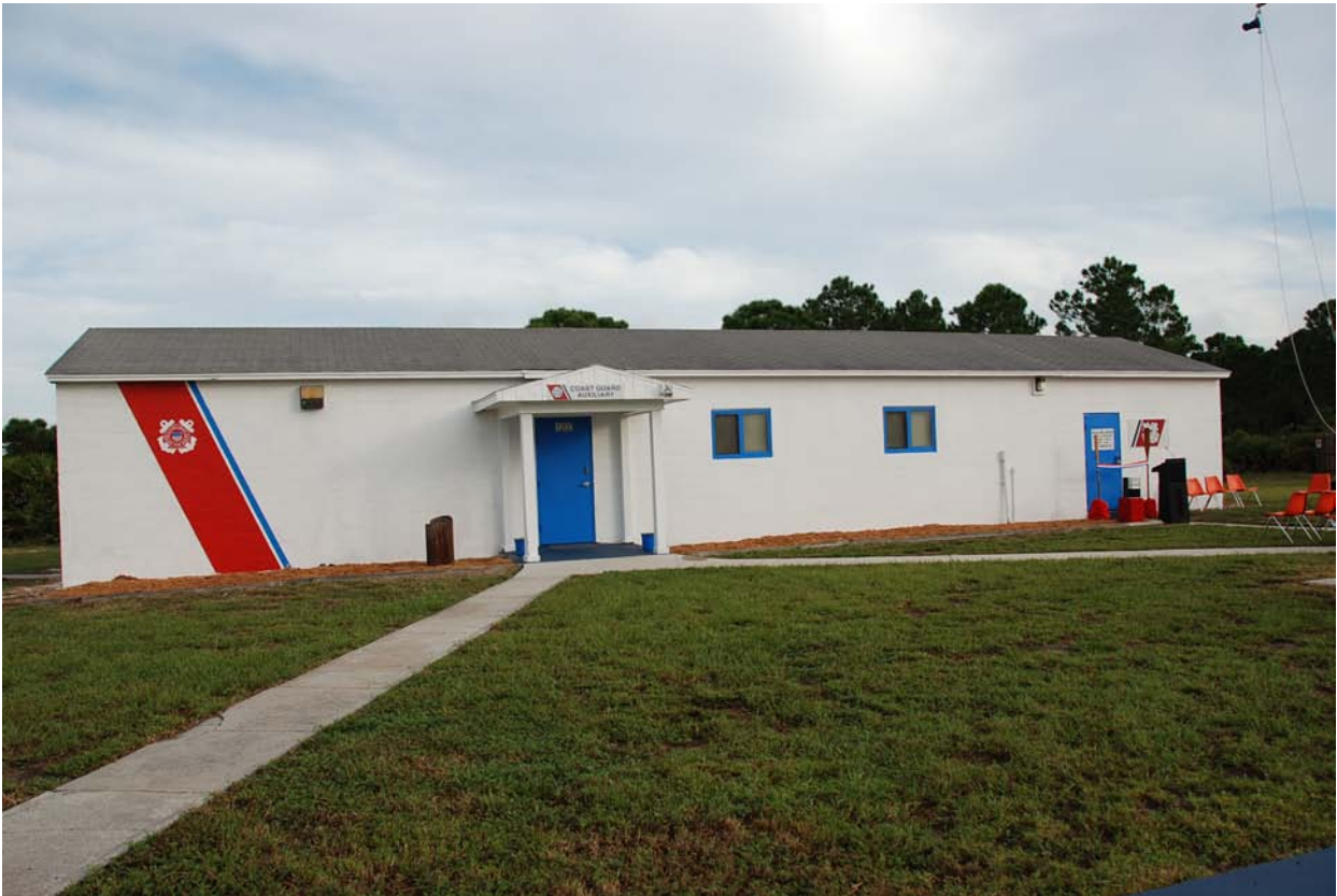
The newly painted Flotilla 86 Training Center which houses Venice Detachment
